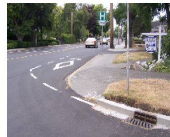
Victoria has painted lane striping at corners that may discourage drivers from running over markings.
